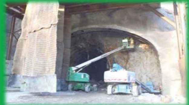
During Widening (Tunnel Width 16.2m)
