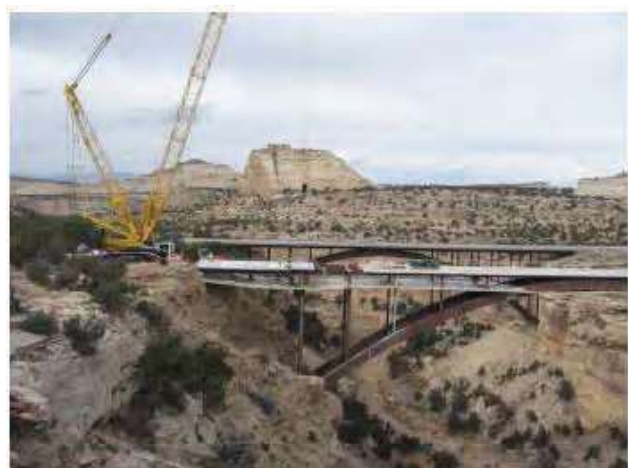
Eagle Canyon Bridge Project
