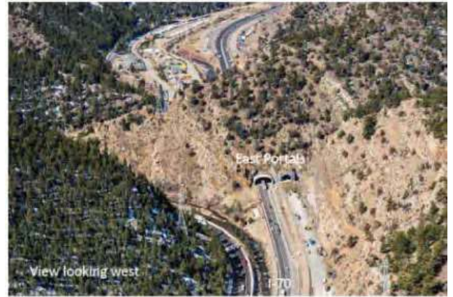
During Widening (Tunnel Width 16.2m)
