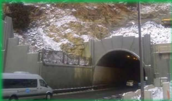
Before Widening (Tunnel Width 9.7m)
