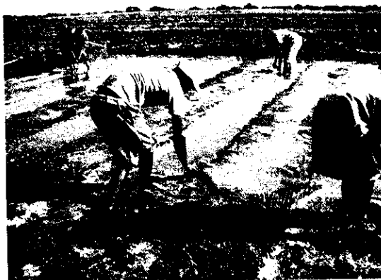
4. Final leveling after putting
