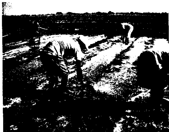
Photo 7. Final leveling after putting water.
