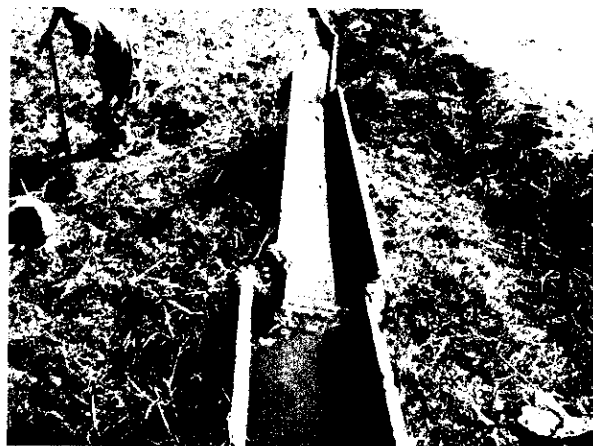
Tertiary irrigation canal (U-flume) was damaged.
