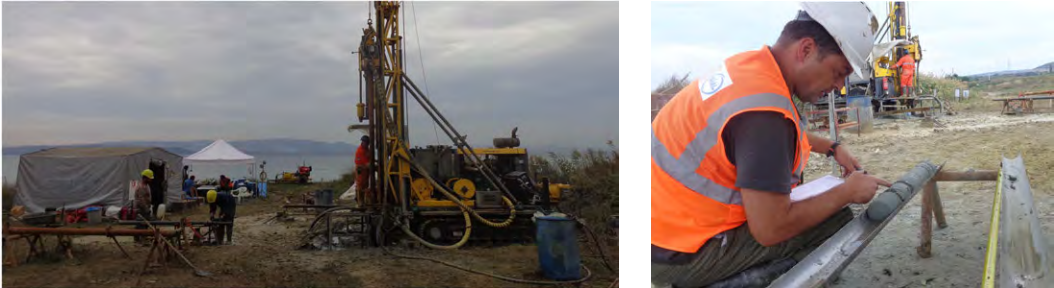
Figure 3.3.15 Drilling and Core logging operations
