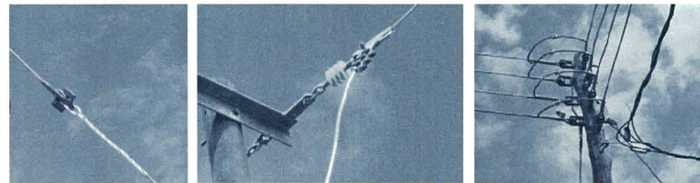
Stay insulator MV tension clamp LV pole fitting
