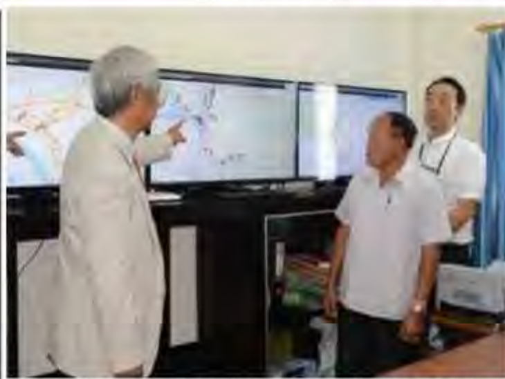
Officials from the concerned organisations visit the CBS office to see the system display installation.
