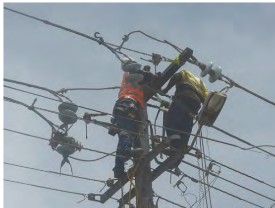
(C) Work on pole
