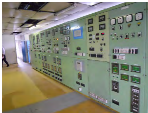
SCADA system in the Taraka substation Control room of the Taraka substation
