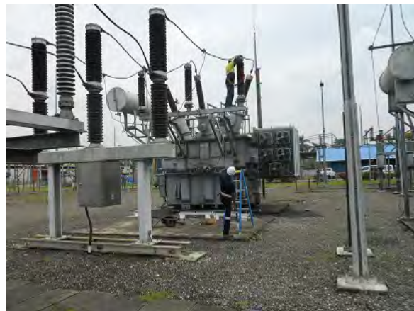
Fig. 2.4-7 Replacement of Arresters
