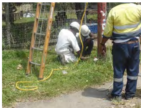
(B) Implanting ground rod
