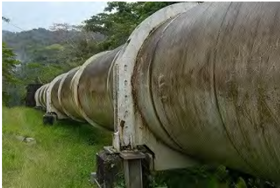
Deformation of the saddle-fixed portion
