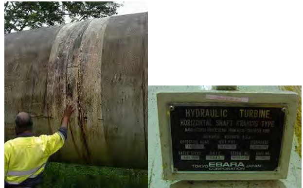
Repaired portion of deformed penstock
