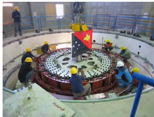
Refurbishment works of Ramu 1 Hydropower plant
