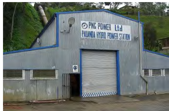
Pauanda Hydropower Plant
