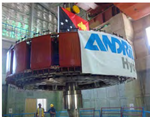
Refurbishment works of Ramu 1 Hydropower plant
