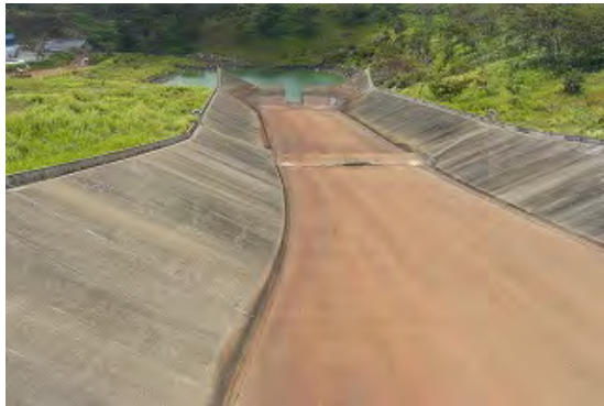
Yonki dam: Spillway
