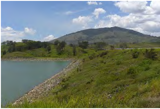
Yonki dam: Upstream view
