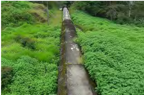
Upper concrete lining portion: Penstock
