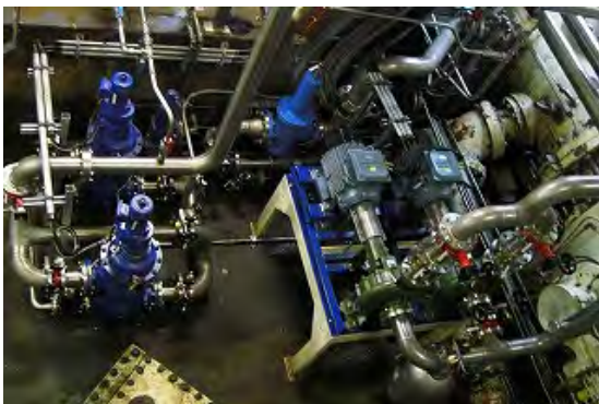
The water cooling system was replaced (Units #1, #2 and #3).
