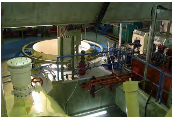
Additional Surge Chamber to be connected to the open penstock
