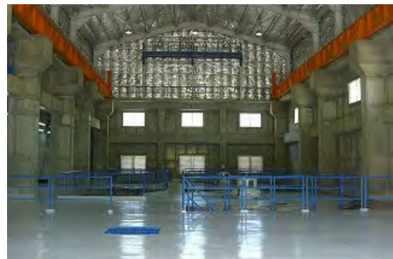
Powerhouse Building 1st floor
