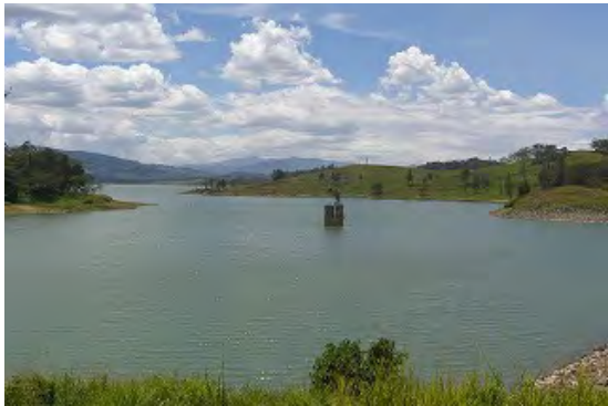
Yonki reservoir dam and Intake tower gate
