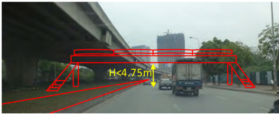
Figure 5.2.9 Not Sufficient Clearance Height under Pedestrian Bridge
