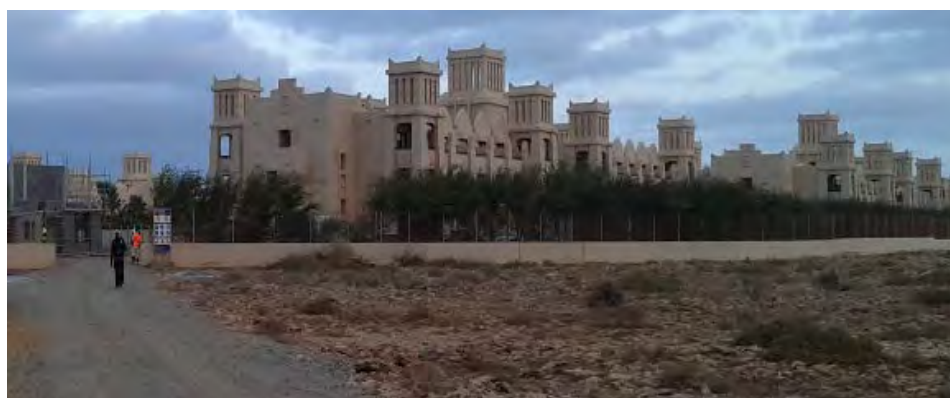
Figure 9.1-16 Resort hotel under construction in the southern region
