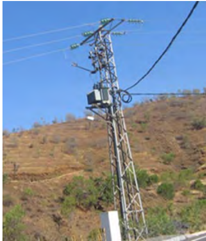
Figure 9.1-2 Pole-mounted and ground-mounted transformers
