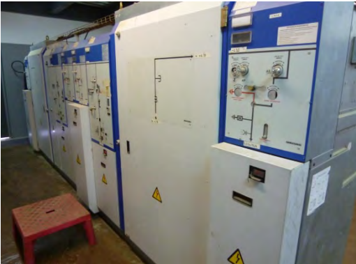
Figure 9.1-3 Switchgears (left: made in out modeled Portugal, right: made in new-style Spain)
