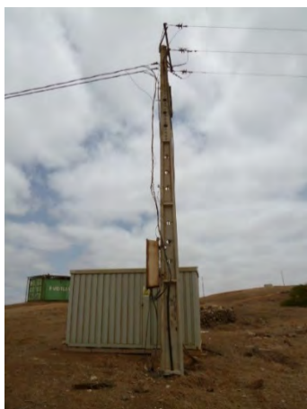
Figure 9.1-14 Connection point at C.d.Tarefes (stationary 25kVA transformer is housed in the container)
