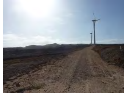
Land utilization conditions (Wind turbine of Vestas 850kW × 3 units)
