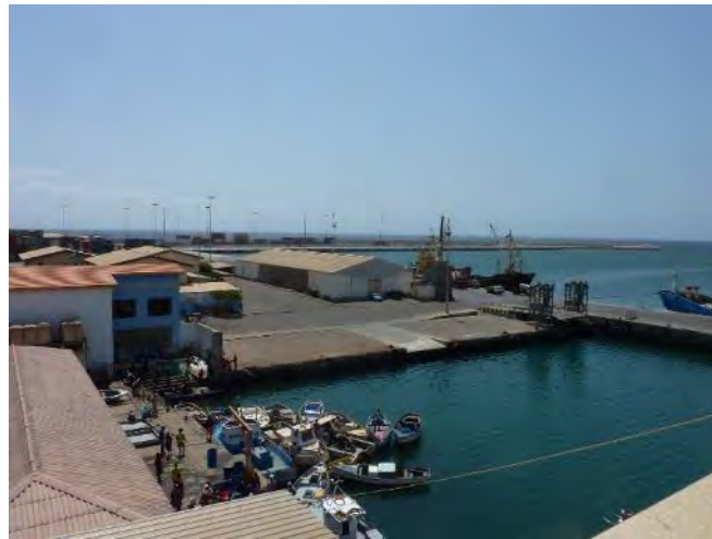
Condition of the wharf at Praia Port (Santiago)
