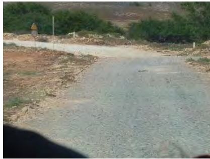
Unpaved road that leads to the power plant premises
