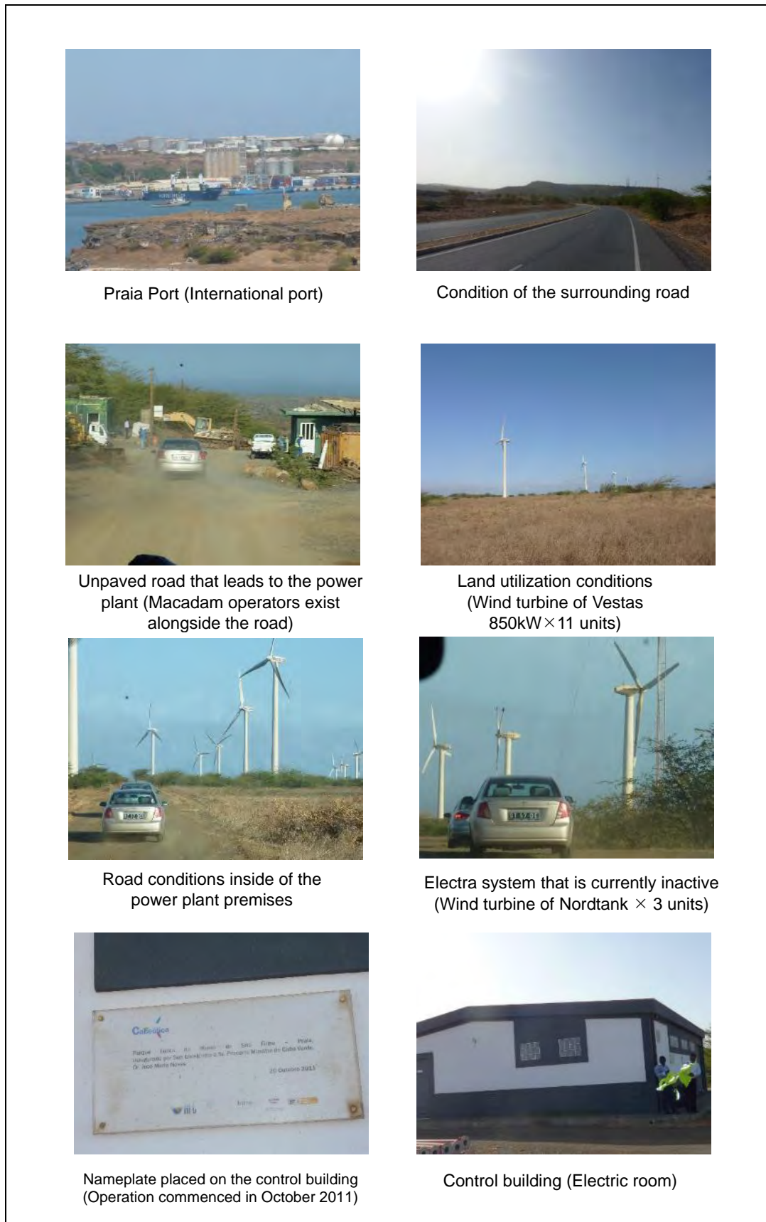
Figure 7.1-2 Conditions of the Santiago wind power generation system
