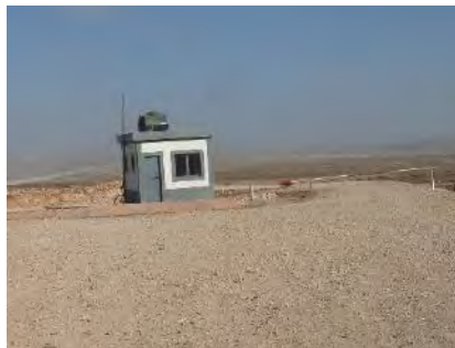
Entry guard station and entry gate inside of the power plant premises
