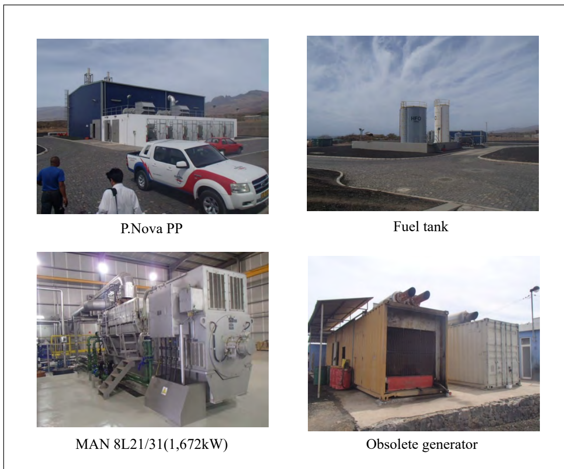
Figure 6.1-1 Diesel power facilities of Santo Antão
