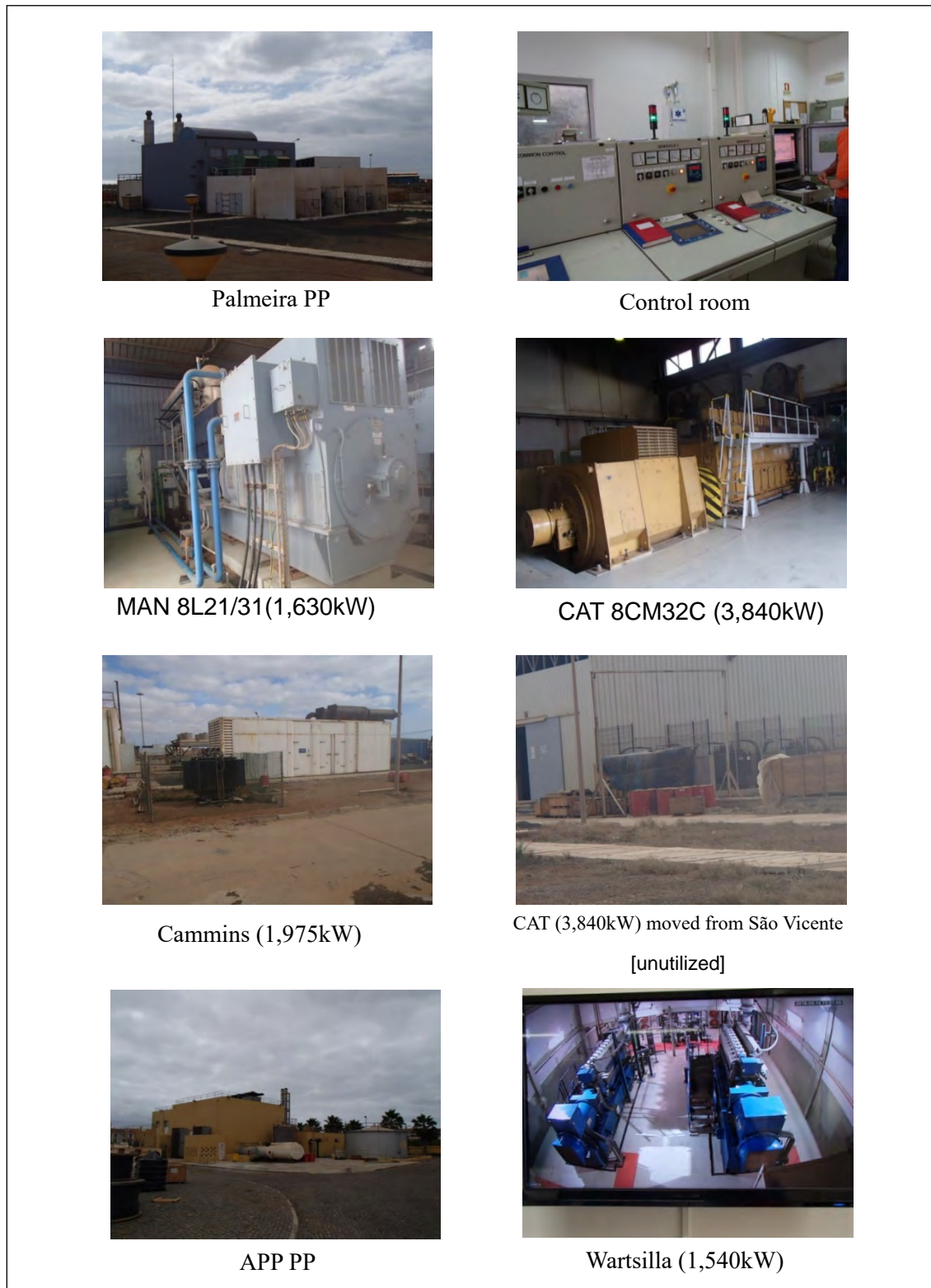
Figure 6.1-4 Diesel power facilities of Sal
