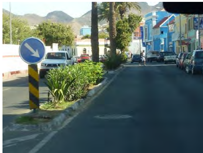
Condition of the road near the Mindelo Port (São Vicente)
