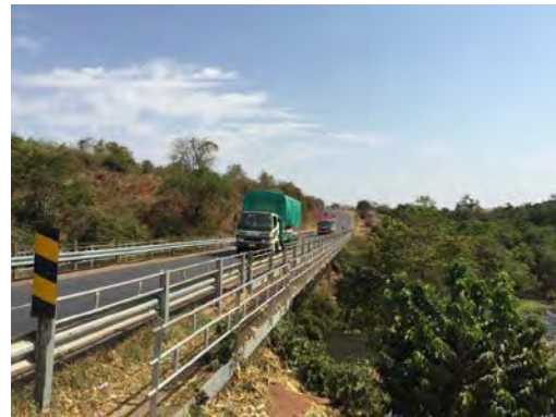
Existing Kikafu Bridge
