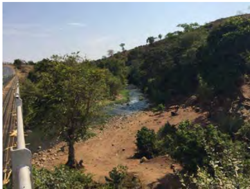
Existing Kikafu Bridge (view of downstream side)
