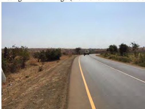
Existing approach road to Kikafu Bridge (Moshi side)
