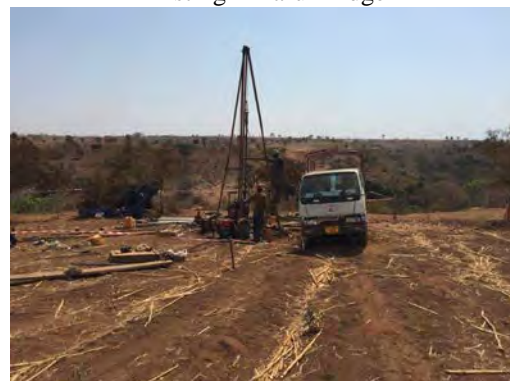
New alignment section (geotechnical boring)
