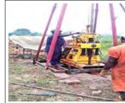
XY 200 rotary drilling rig mobilized for the ground investigations
