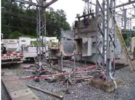
Figure 7-12: Example of damage caused by a snake at a substation
