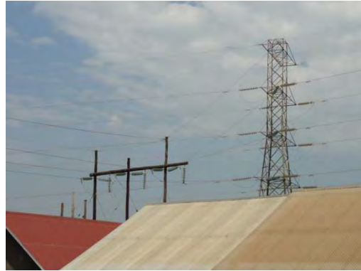
Photo 3-2-4.2 Transmission line between Kampala North Substation and Mutundwe Substation (Left: 132 kV wooden poles to Kawaala Right: No.570 tower)
