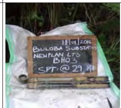
SPT at 29m for BH3, very dense reddish yellowish grey silt of high plasticity, elastic silt
