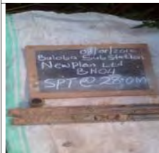
SPT at 28m for BH4, moist mottled greyish brown firm intact silt of high plasticity, elastic silt
