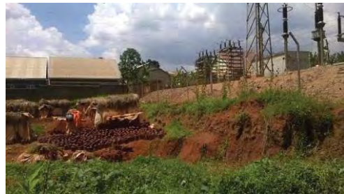
Figure 7-8: Showing proximity of houses to Kawaala SS fence line
