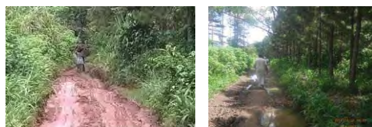
Figure 7-5: Narrow and rutted sections of the access road to the substation site
