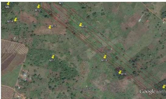
Figure 3-21: Mukono - Transmission line closer to West end
