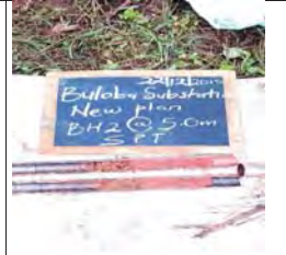
SPT at 5m, moist reddish brown stiff intact silt of high plasticity, elastic silt
