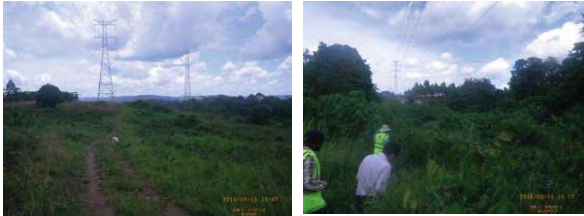
Figure 7-6: Transmission lines to the extreme North (Left) and to the extreme South (right) of the proposed route
