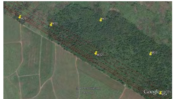
Figure 3-19: Mukono - Transmission line traversing Nandagi Forest Reserve
