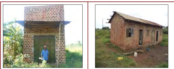
Photo 2: Example of structures that will be affected by the transmission line
