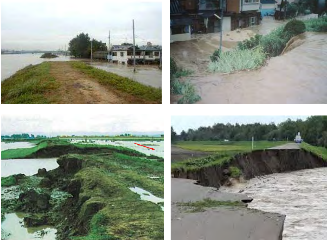
Figure 3-2 Destroyed Dyke due to Overflow and Erosion
