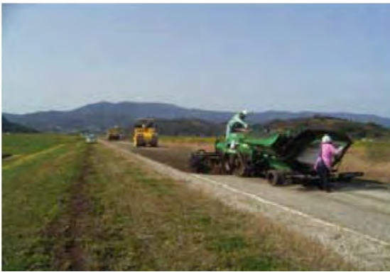
c) Repair of Dyke Crown
