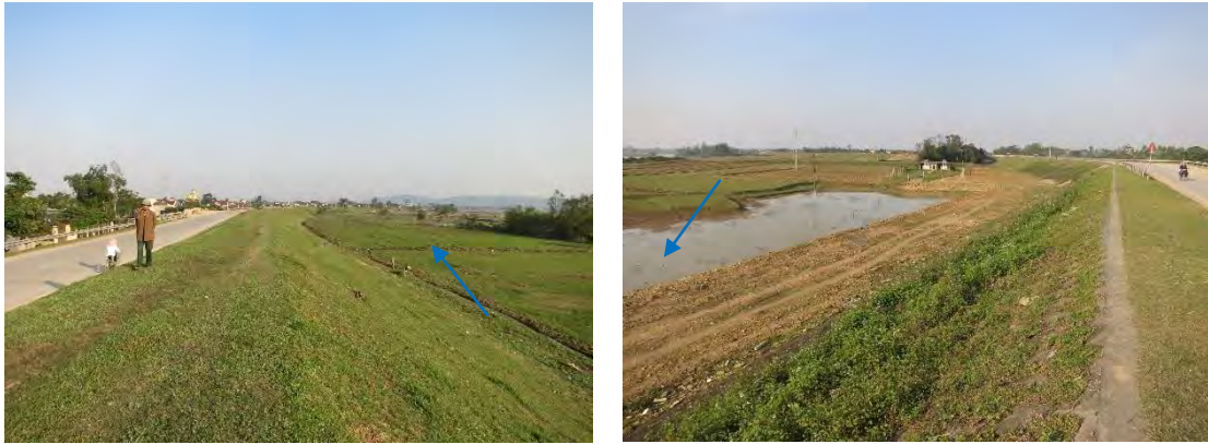
Figure 4-3 Well Trained Dyke in Ca River
