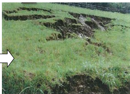
d) Erosive expansion due to Rainfall
