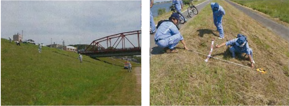
Figure 4-2 Dyke Inspection by Patrol
