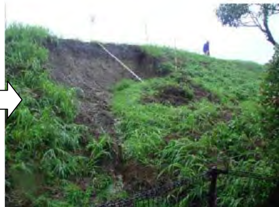
b) Slope Failure immediately after Flooding
