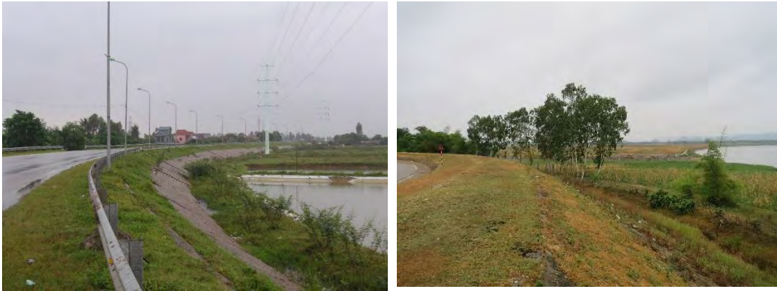
Figure 2-2 Existing Dyke in Lower Ca River (Lower Reach: Lam River)
