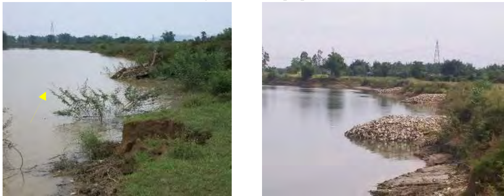
Photo 3-4-2 Before / After of construction in Ha Tinh province (Series of 6 groins)
