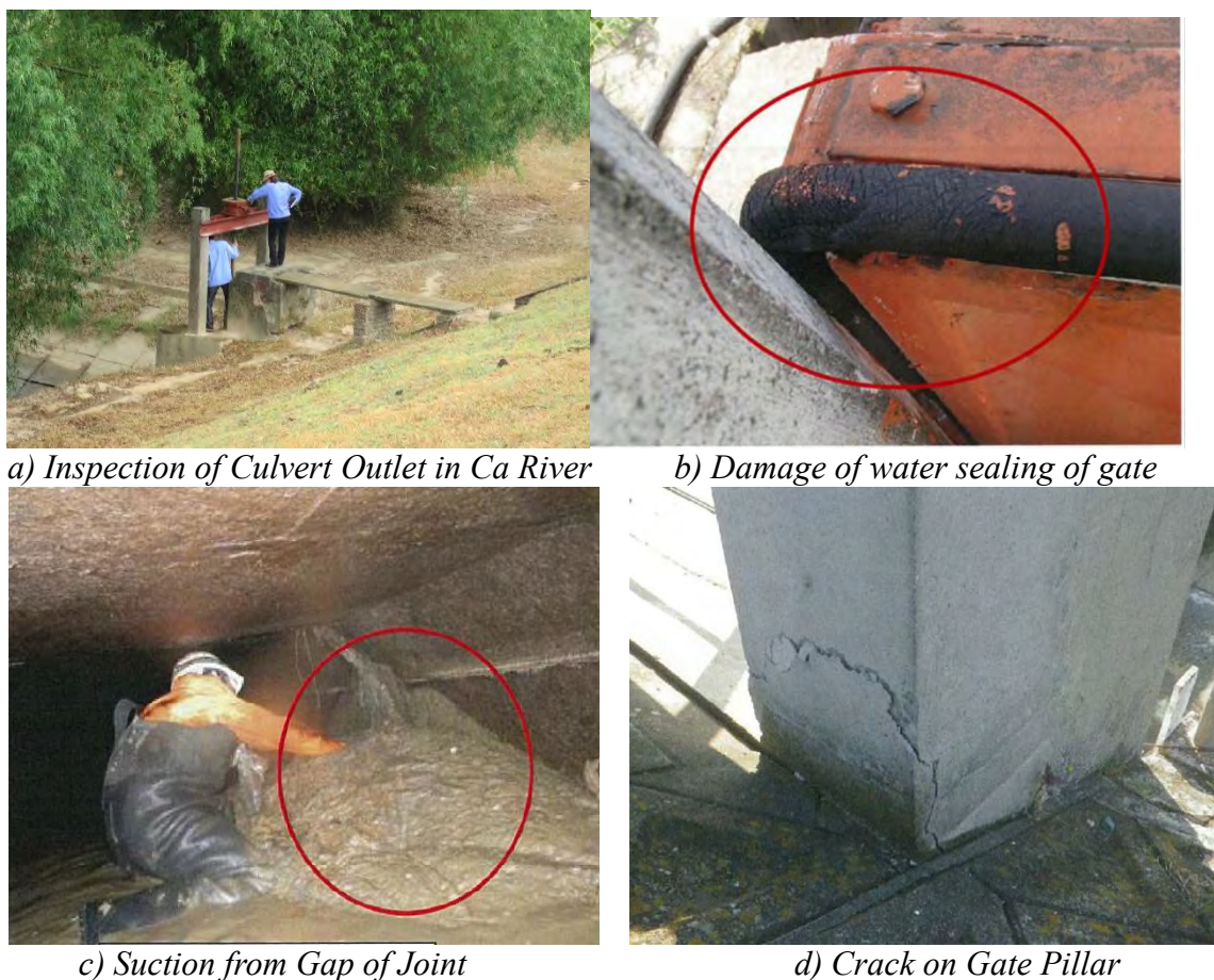
Figure 4-12 Inspection of Culvert Outlet/Groin
