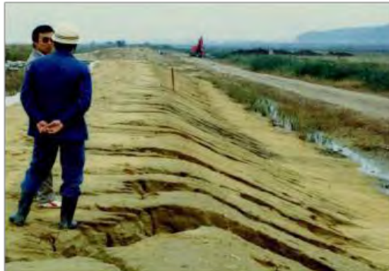
(Data source: Dr. Uno, Gifu University, Aug.2010) c) Erosion (Gully) due to Rainfall
