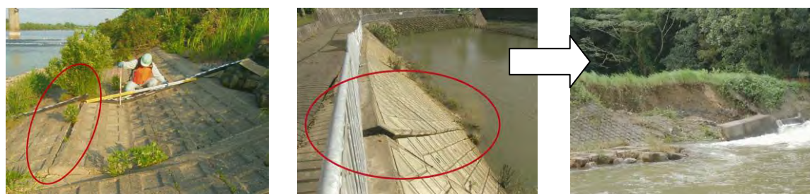
Figure 4-13 Inspection of Riverbank Protection Works
