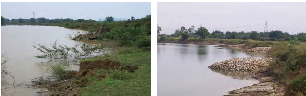
Fig 18 Before and after the construction of groyne in Hà Tĩnh
