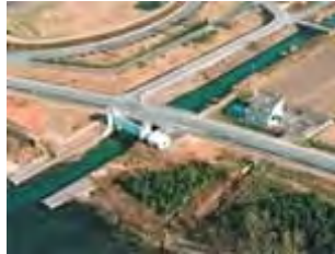
Drainage pump station
