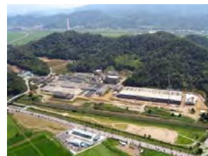
Tohoku-bu Sewage Treatment Plant
