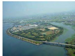
Konan-chubu Sewage Treatment Plant
