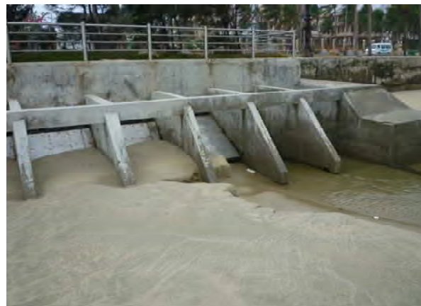
Photo 4.2 Outfall on the beach after high tide period
