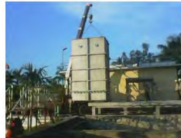
Construction U-BCF at Vinh Bao (August 2013)
