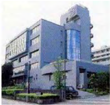
Source: Japan Sewage Works Agency Picture 4.3.1 Multipurpose Practice Building
