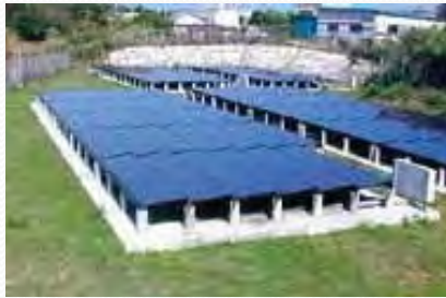
Survey, planning, and construction work management of 200 kW PV project in Kita Daito Island
