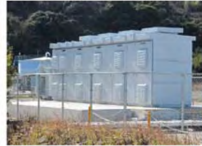
Self-standing Outdoor Type (250kW x 4)
