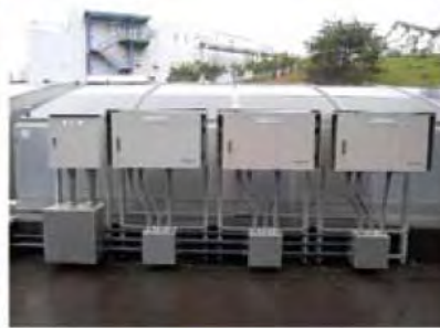
Wall-hanging Outdoor Type (10kW)
