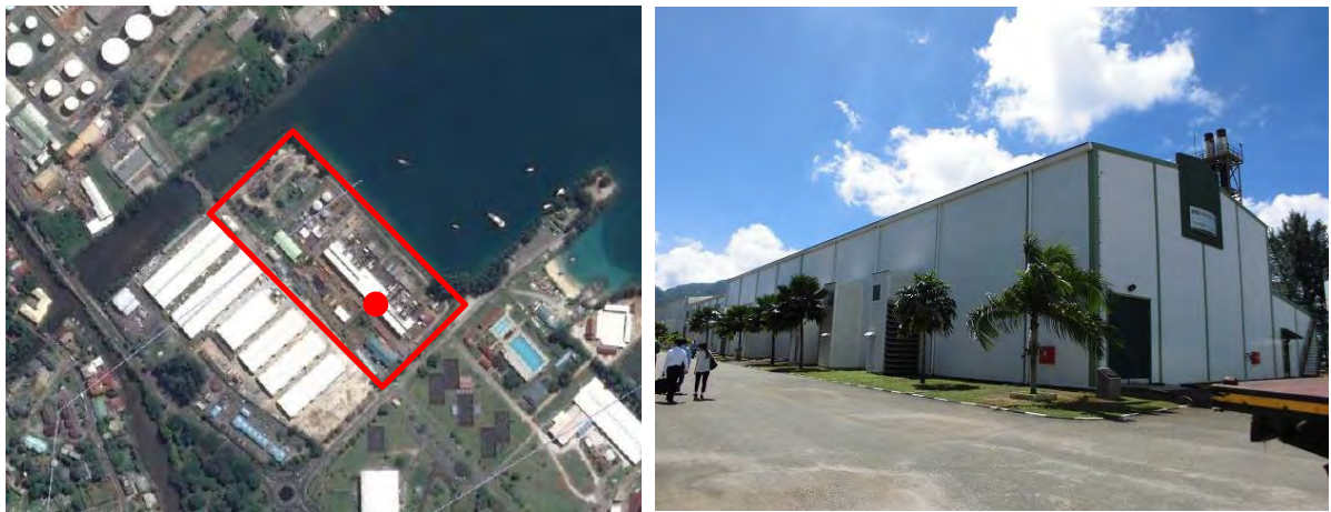
Victoria C Power Plant premises
