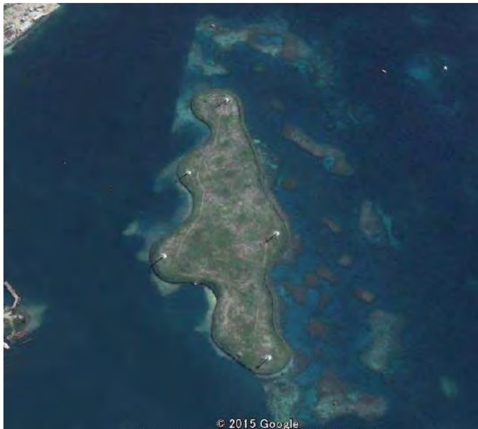
Figure 3.3.3-1 Islands with wind turbines installed
