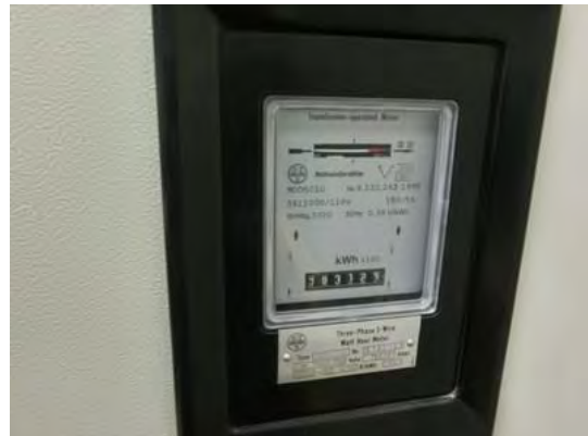
Figure 3.2.5-15 Electricity meter (SET 6P-8P)
