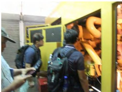
Power plant survey conditions (Desroches Island)
