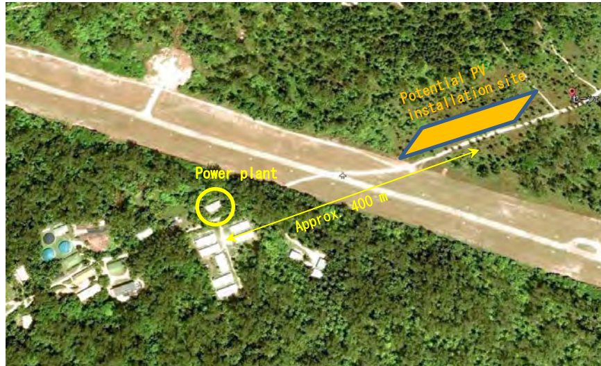
Figure 2.5.3-3 Diesel power generation facility and potential installation site for PV facility
