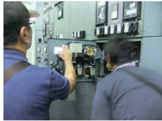
Measurement signal extraction survey (Praslin Island)
