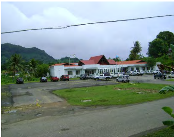
Target site north side (Kosrae State government building)
