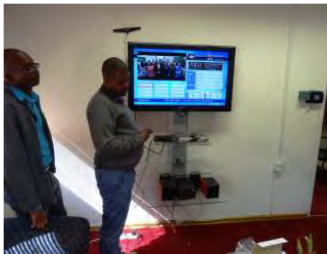
Installation of receivers for demonstration (June, 2015)
