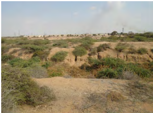
Proposed coal stockpile site to the east of NWIZ. The stockpile is planned up till the fence of PSM which is visible in the background along with PSM buildings. The westward water channel flows through the center and has eroded the land around its banks.
