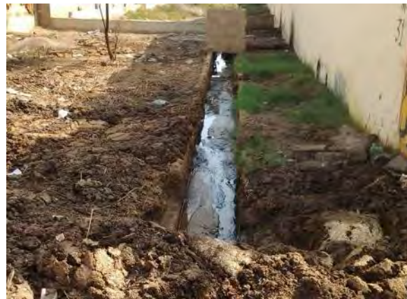
Direct discharge of effluent into open drains
