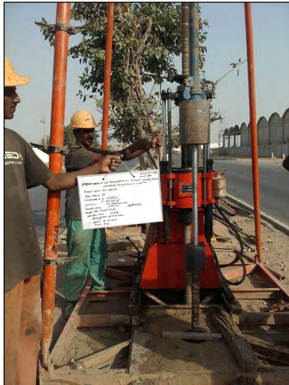
BORE HOLE NO. 10
