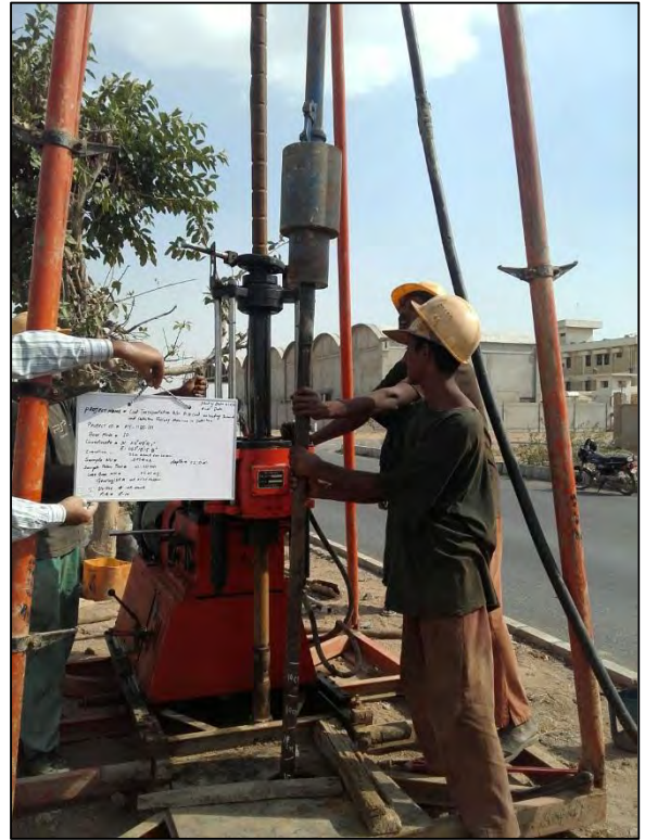
BORE HOLE NO. 10
