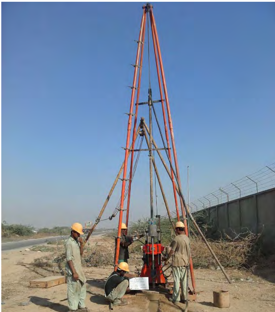
Figure A-1 Drilling works in progress
