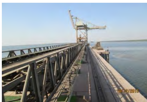
Figure 4-5 IOCB Jetty and Unloader and Conveyor Belt on Trestle
