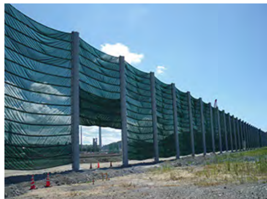
Figure 4-18 Stacker Reclaimer and Dust Suppression Net
