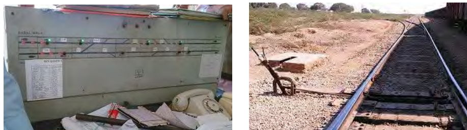
Figure 6-3 Temporary Signaling Control Panel and Manual Point Machine
