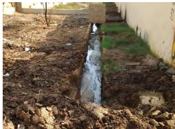
Direct discharge of effluent into open drains
