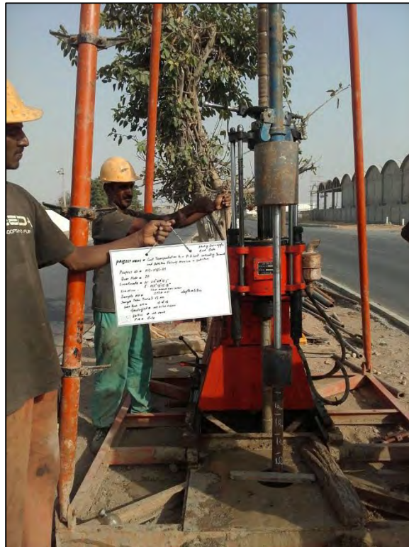
BORE HOLE NO. 10
