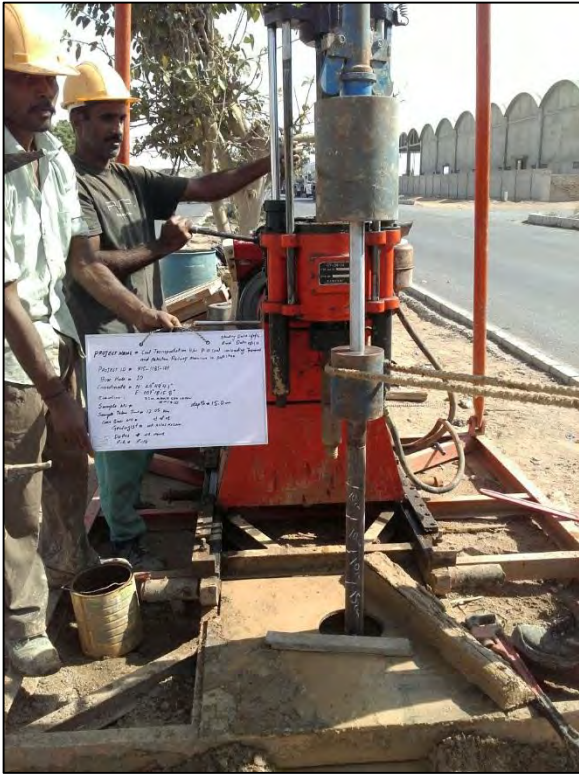
BORE HOLE NO. 10
