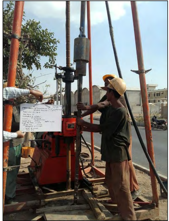
BORE HOLE NO. 10
