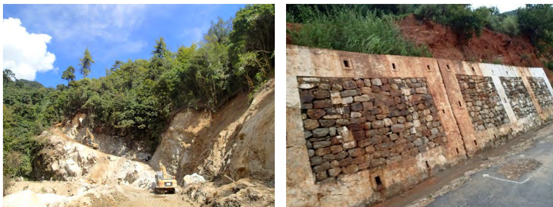
Figure 6.1.2 Photo of Typical Countermeasure Works in Bhutan, Excavation Work (left), Masonry Retaining Wall (right) (Source: JET)
