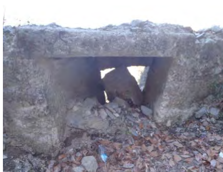
a) Soil and boulder in the culvert (WPP0120330)
