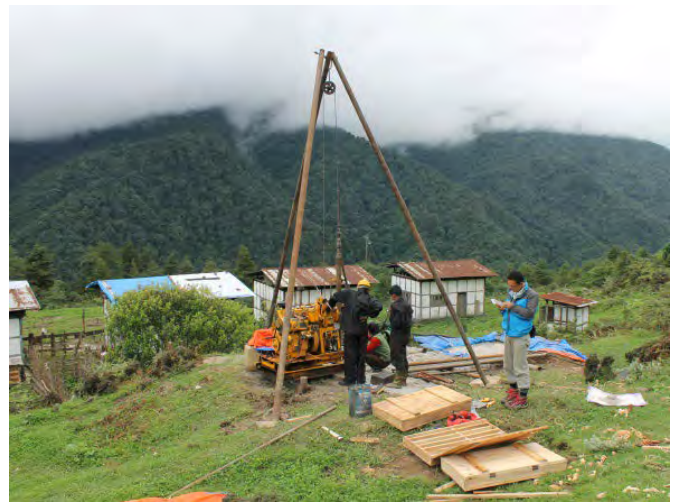
Drilling works, Bangla Pokto Area, June 2015
