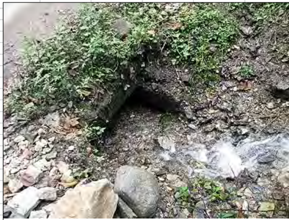
Close view of the inlet
