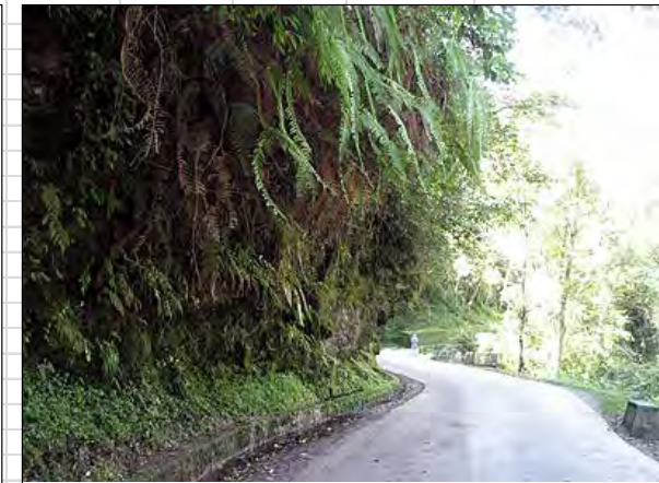
Close view of overhung rocks at end point
