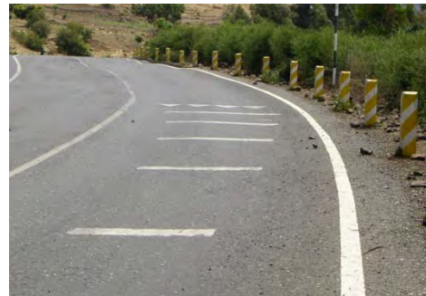
Figure 2.4.12 Photo of the Sign on Road to Notify Corrugated Road Surface on Ahead (Source: JET)
