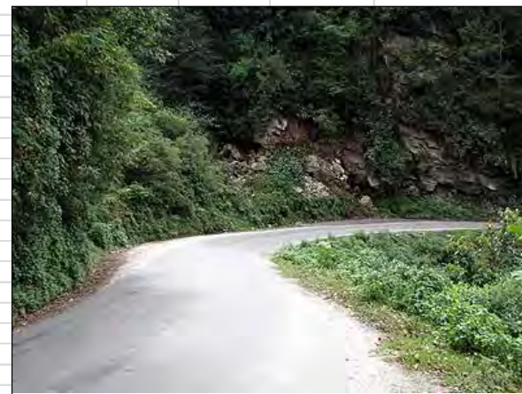
Clearance between road and the debris from start side
