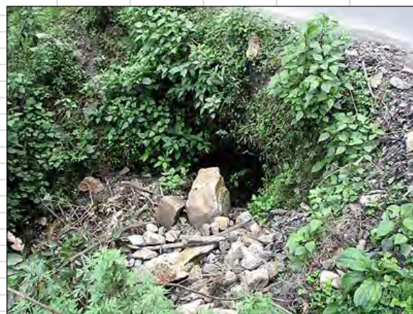
Close view of the outlet
