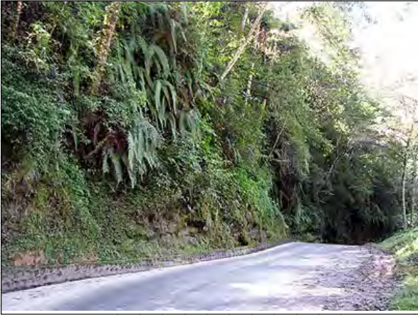
Full view of the slope at start point
