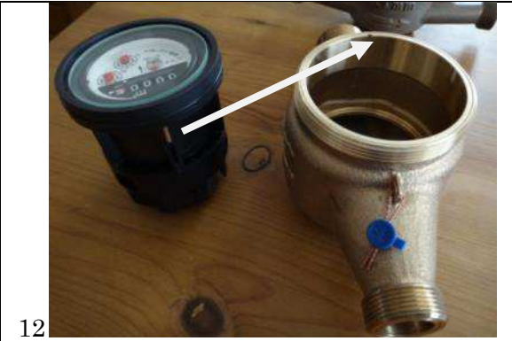
Assemble meter unit & iron case
