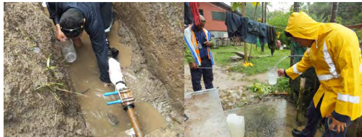
Figure R-1 Measurement of Leakage Volume
