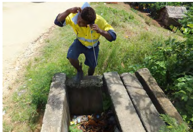
Figure 6.4-2 Leak sound checked by using Listening Stick
