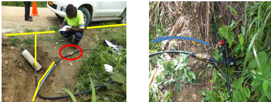
Figure 4-9 Measurement for Separation of Service Lines
