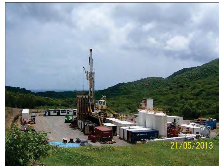
Figure 11: Typical Layout of Geothermal Drill Rig and Pad (in Montserrat)
