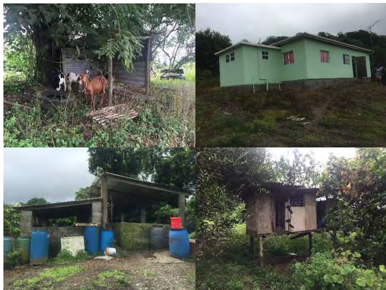
Figure 52: Residential and Farm Structures on Site W3.
