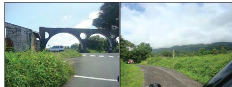
Figure 42: Orange Hill Aqueduct (L) & “Feeder” Road to Sites W1 & W3 (R)
