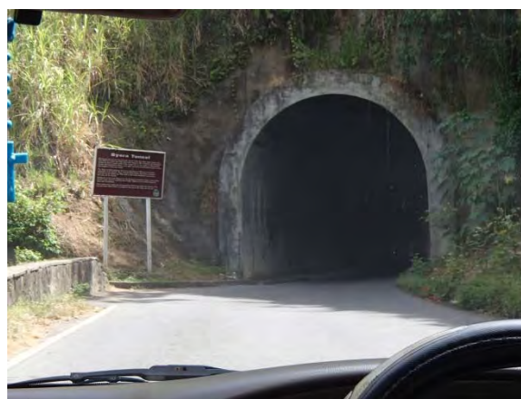
Byera tunnel located at the eastern coastal road
