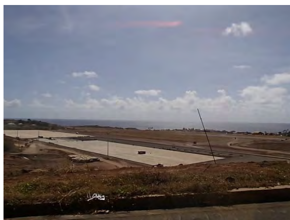
New international airport (under construction)
