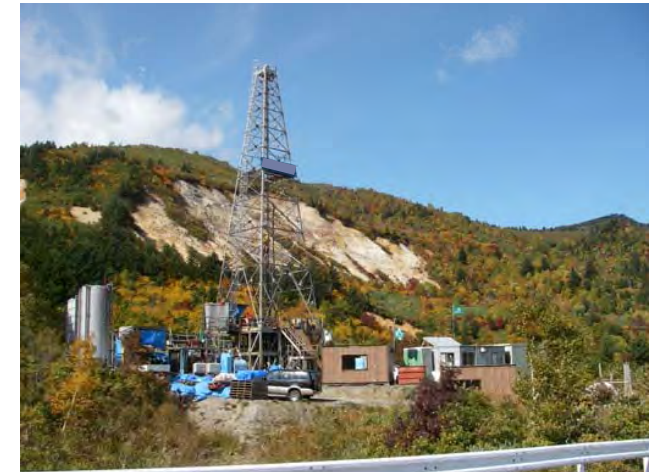
Drilling rig for slim hole 2000m Hachimantai, Japan Source:JICA team
