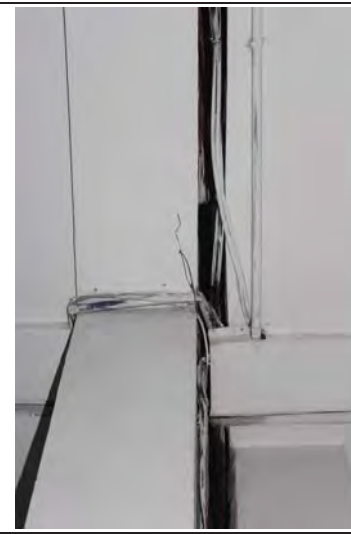
Narrow expansion-joint
