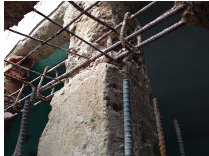
Reinforcing-bar arrangement in existing beam
