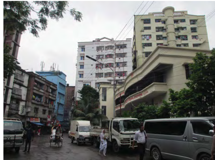
Road in front of fire station
