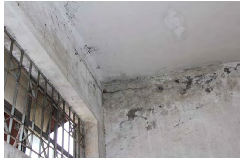
Corrosion of existing reinforcing-bar in beams
