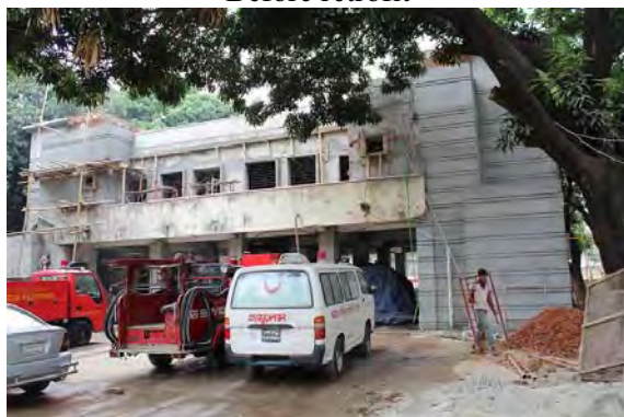
Recent construction site
