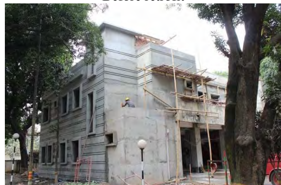
Recent construction site
