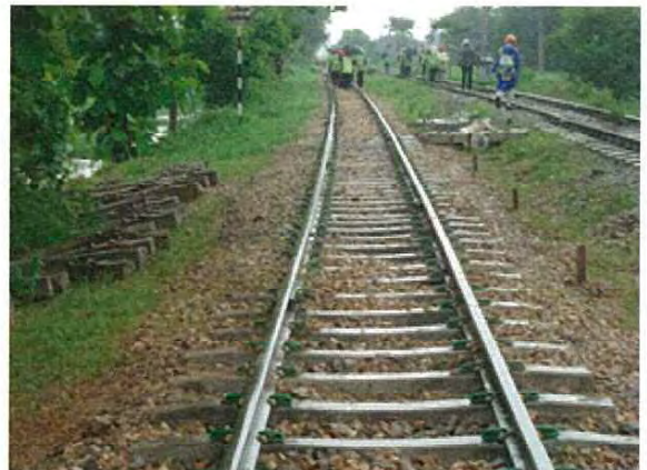
After replacing sleepers
