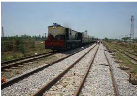
Reverse direction operation under track closing
