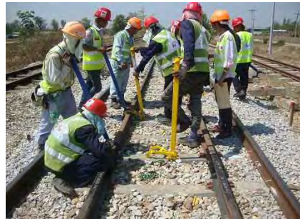
Installing fastening (First Clip)
