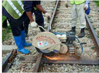
Cutting a rail
