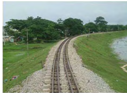
Embankment near Aungthuhka Sta.(2015)
