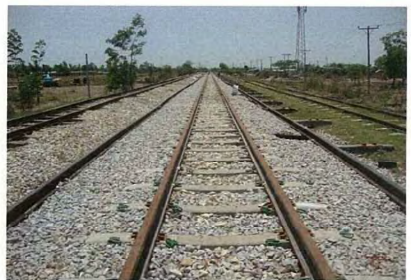
After changing from 75lb rail to 50N Rail
