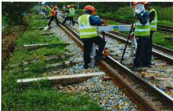
Removing 75lb Rail
