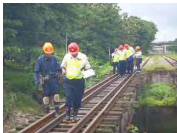
Inspection training on No9 Br
