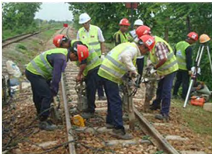
Tamping by hand tie tamper
