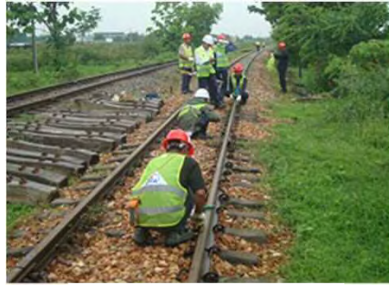
Chord-to-rail measurement
