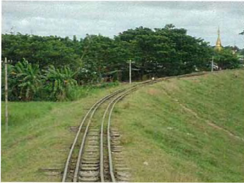
Embankment near Aungthuhka Sta.(2012)
