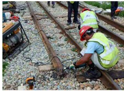
Chamfering (Removing sharp edges)
