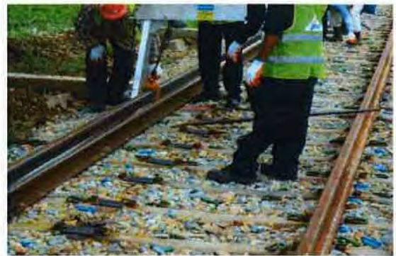
Installing 50N Rail
