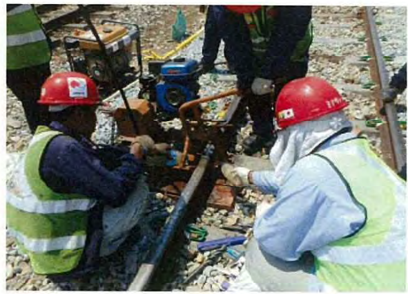
Drilling rail on the trunk line (Pre-Work)
