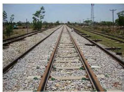
After changing from 75lb rail to 50N Rail
