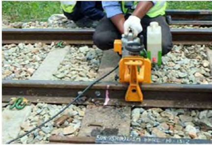
Drilling a hole of the rail
