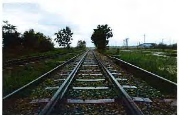
After replacing from 75lb rail to 50N rail
