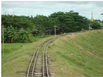
Embankment near Aungthuhka Sta.(2012)
