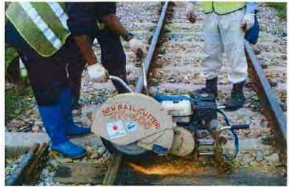
Cutting a rail
