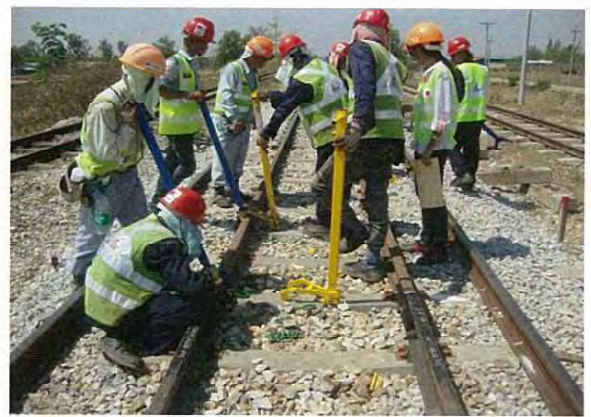
Installing fastening (First Clip)
