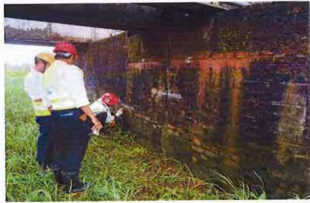
Inspection measurement training follow up
