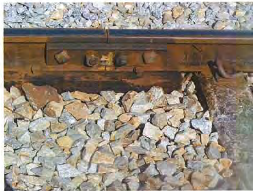
Short sleeper at joint
