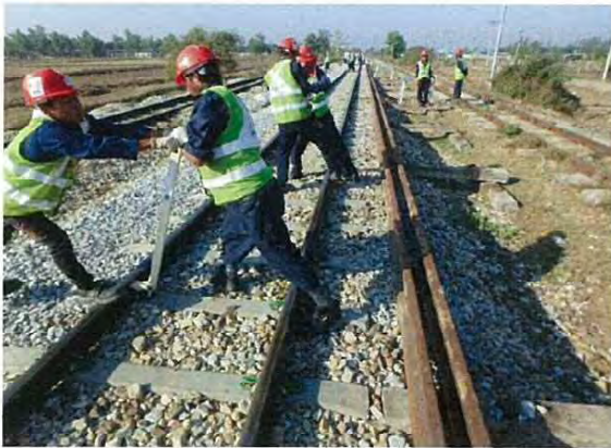
Removal of fastening (Pre-Work)
