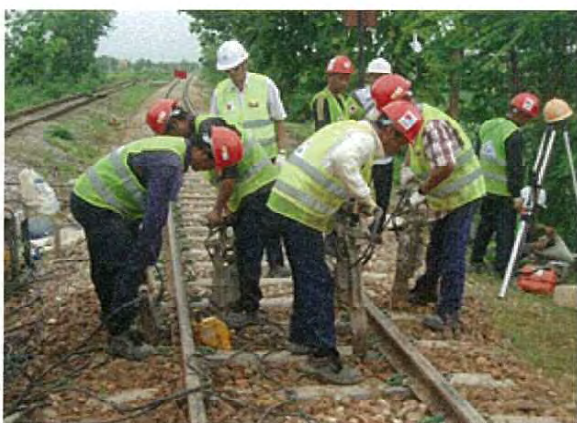
Tamping by hand tie tamper
